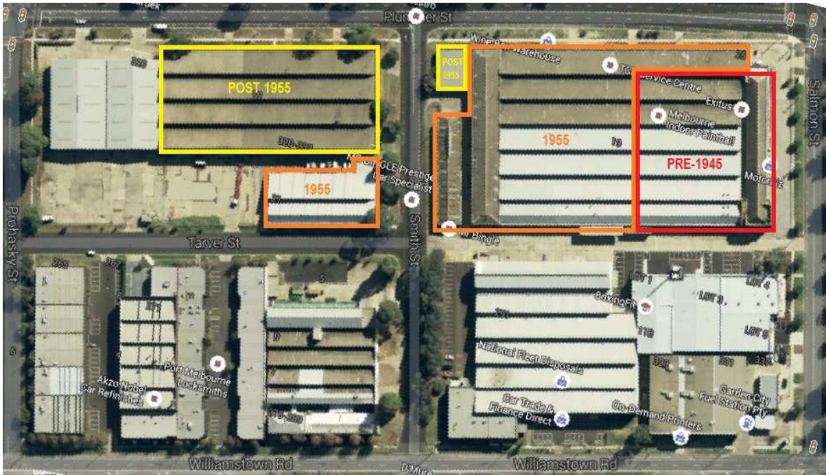
Figure 8 Current aerial photograph, colour-coded to indicate phases of construction: pre-1945 (red outline), 1955 (orange outline) and post-1955 (yellow outline).
