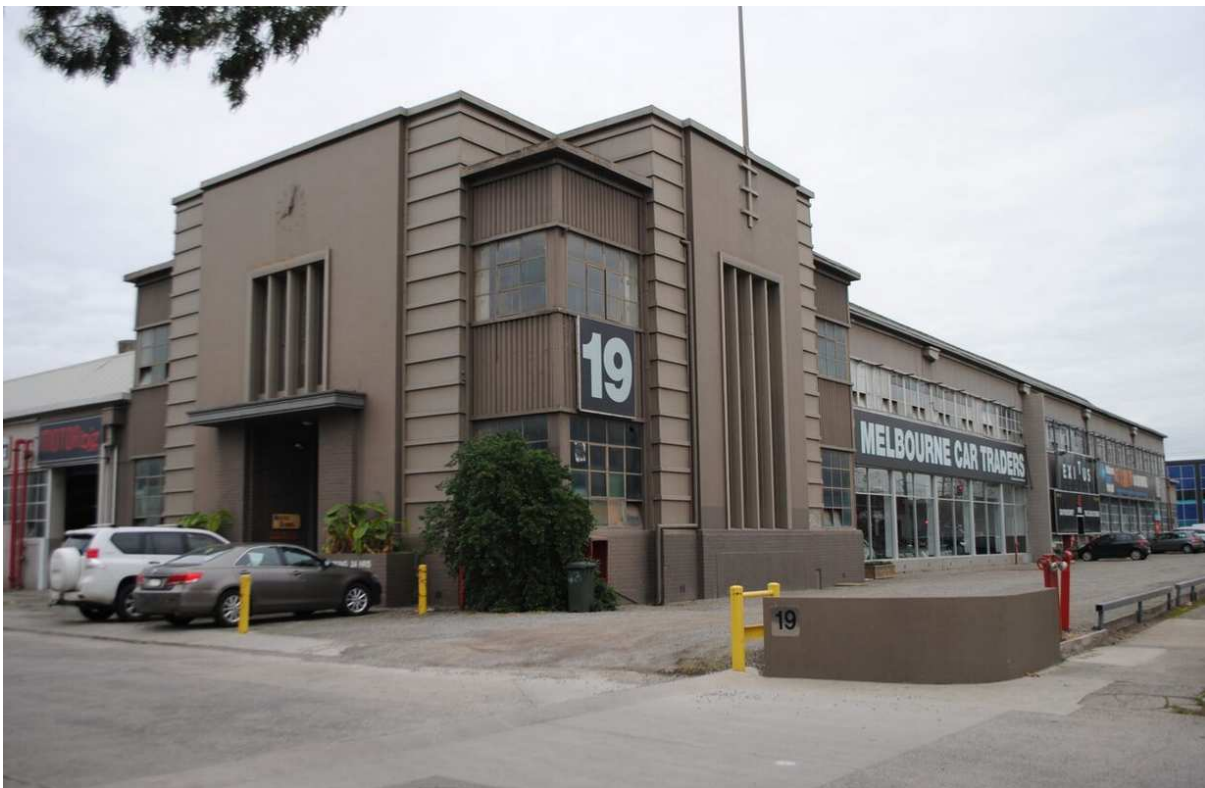
Figure 9: South end of the Salmon Street frontage of administration block, showing entry bay (source: photograph by National Trust of Australia (Victoria), July 2015)
