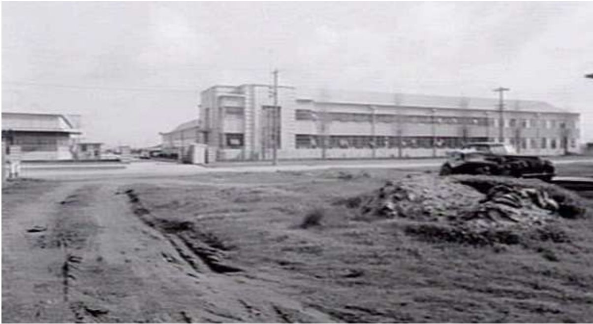
Figure 1: View of the factory during its original governmental occupation, circa 1941 (source Harold Paynting Collection, Picture Collection, State Library of Victoria)
