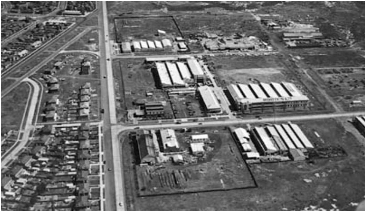
Figure 4: Aerial photograph of the factory, circa 1947, looking west across Salmon Street (source: Item L1849, Series A1200, National Archives of Australia)
