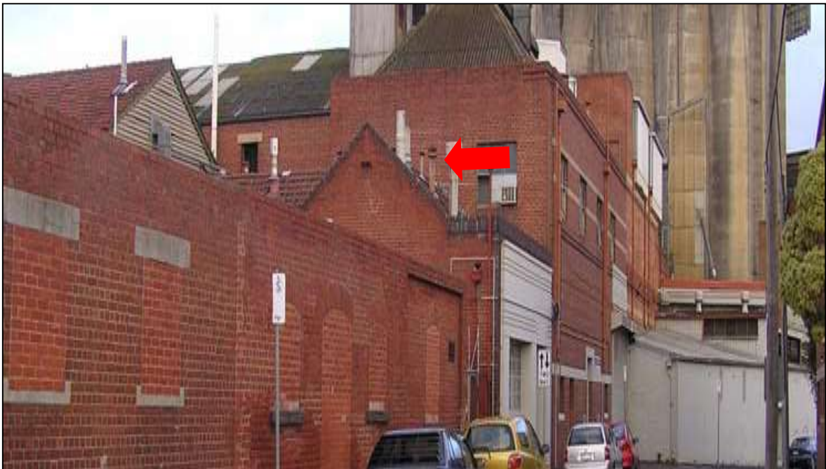
Figure 8 B4, east elevation (indicated by red arrow), as seen from the east on Gough Street; note the former kiln roof towers behind the barrel vaulted ridge vent, to be retained and re clad
