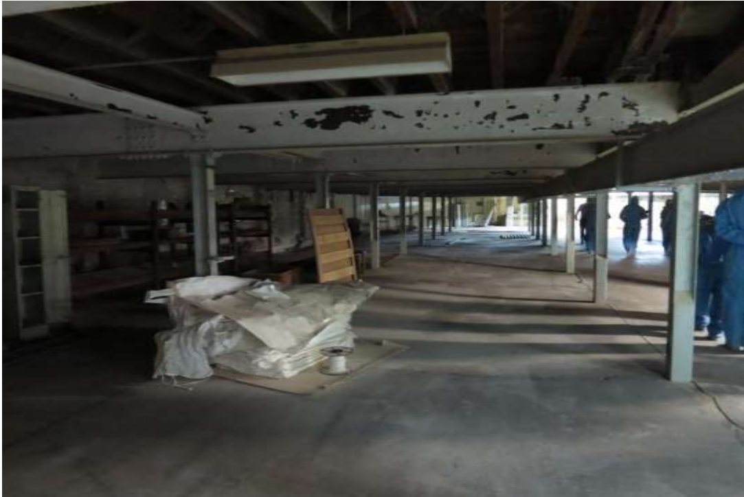
Figure 26 B6 interior, ground floor, showing concrete germinating floor with 'spoon' profile, and regular grid of steel stanchions and girders
