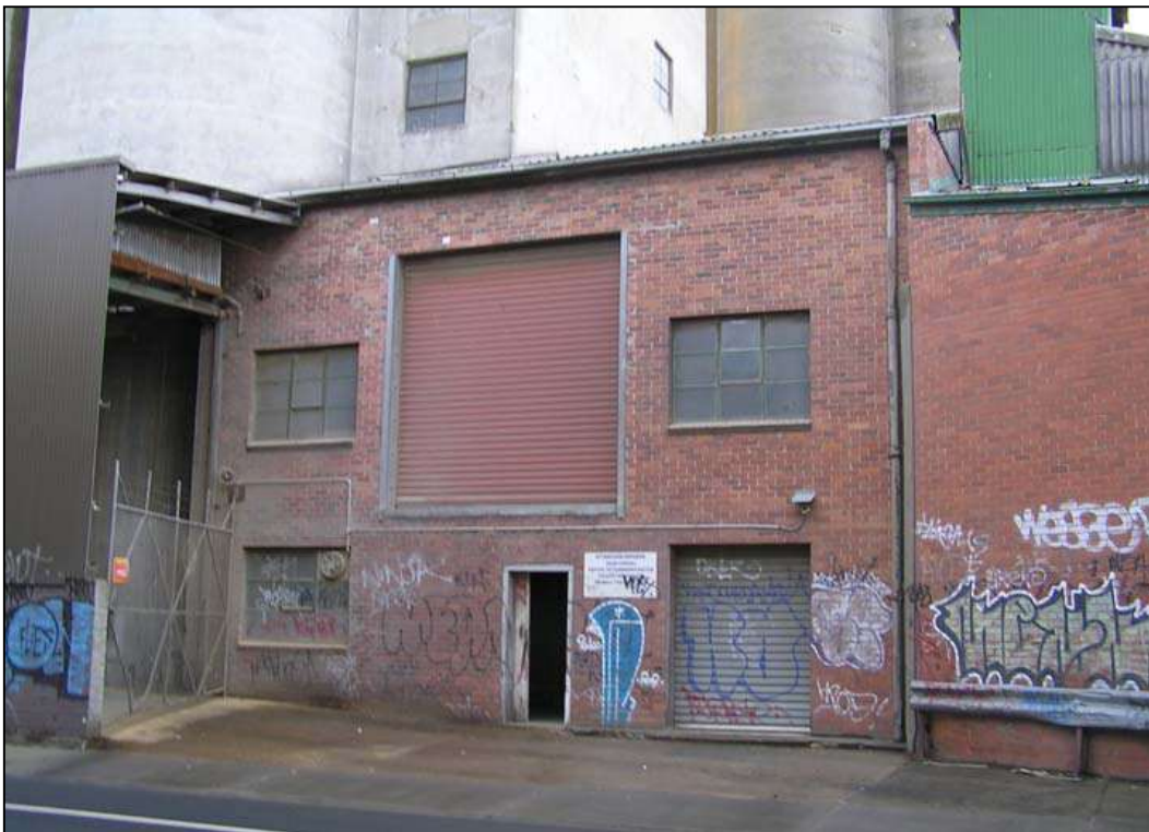
Figure 23 B6, western addition, showing the south elevation to Harcourt Parade; this component is proposed for demolition
