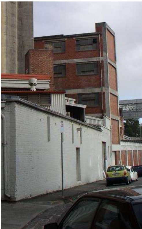
Figure 40 East side of B10 tower
