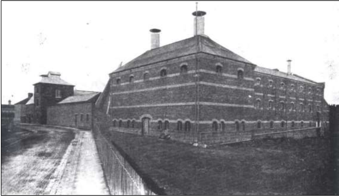
Figure 18 1903 view of Richmond Maltings, on Cremorne Street; the main building in the foreground is the 1880 malt house (B5), with its kiln roof form already modified from the original; the large west elevation at right is proposed to be revealed and restored Source: Australian Brewer's Journal . 20 February 1906
