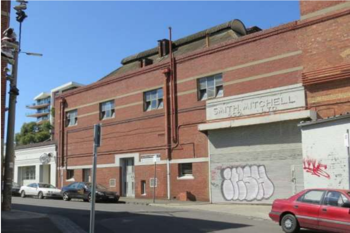
Figure 7 B4, north elevation to Gough Street; the majority of this current form and appearance of the façade will be maintained, as will the barrel vaulted ridge vent to the roof
