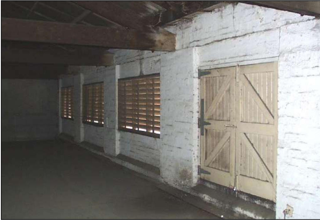
Figure 45 B11, interior of level 2 (top level)
