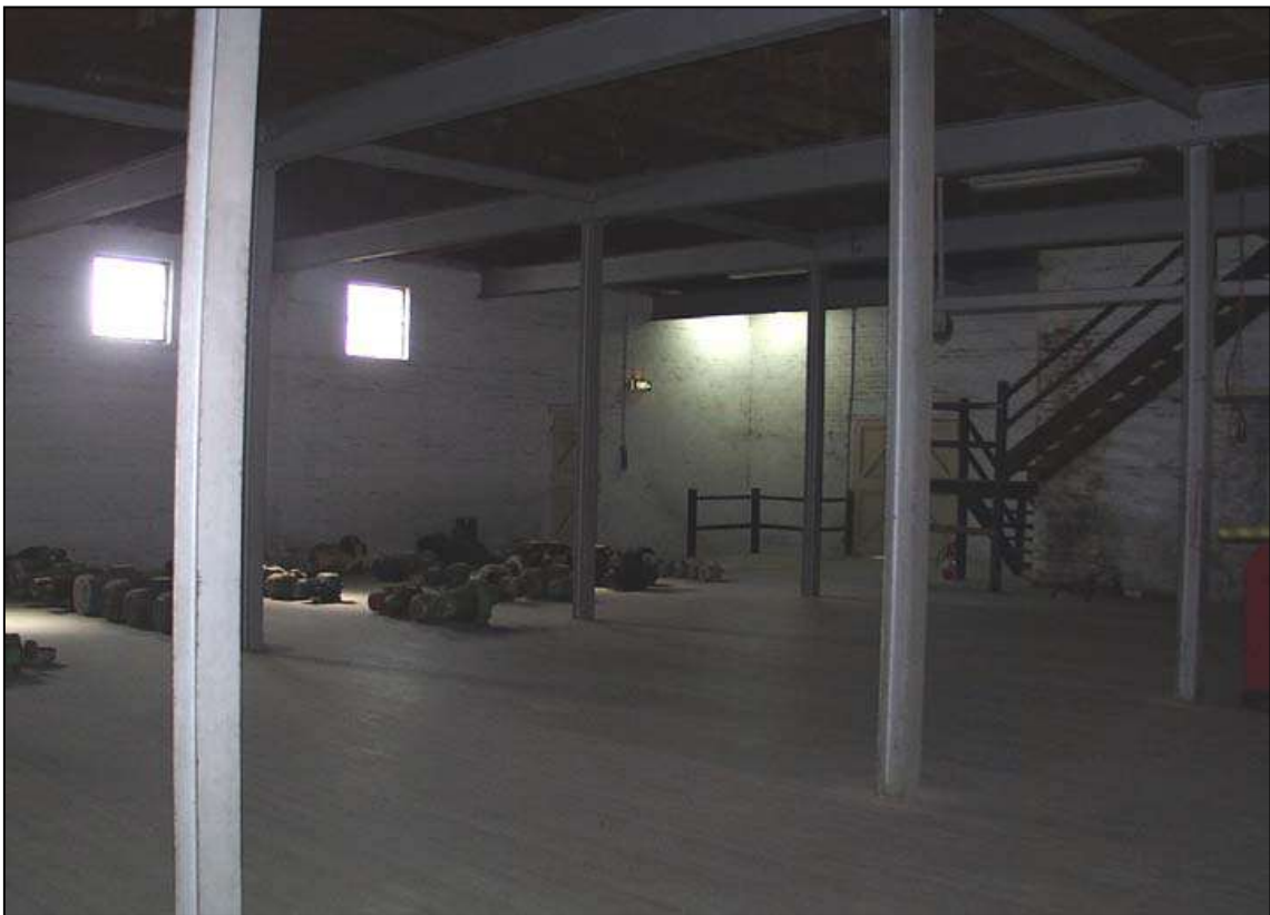
Figure 44 B11, interior of level 1 (middle level)
