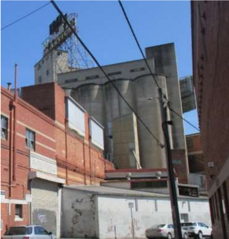
Figure 30 East side of B8 silos, showing concrete cylinders and associated grain elevator tower at right
