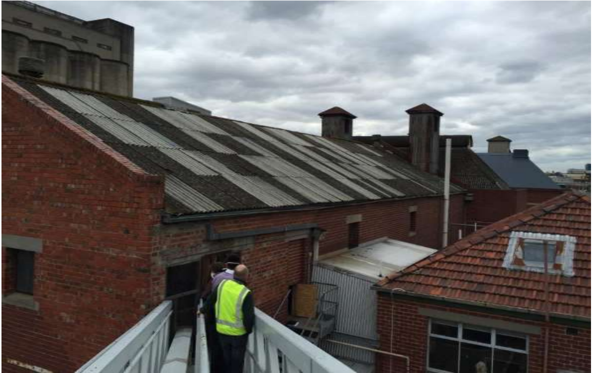
Figure 11 B4 roof with the kiln towers visible, and the south end gable at left; B3 is at right
