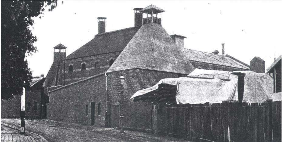
Figure 20 1919 view of Richmond Maltings, on Cremorne Street, showing B5 with the (then new) 1918/19 addition in the foreground Source: Australian Brewer's Journal . 20 January 1919
