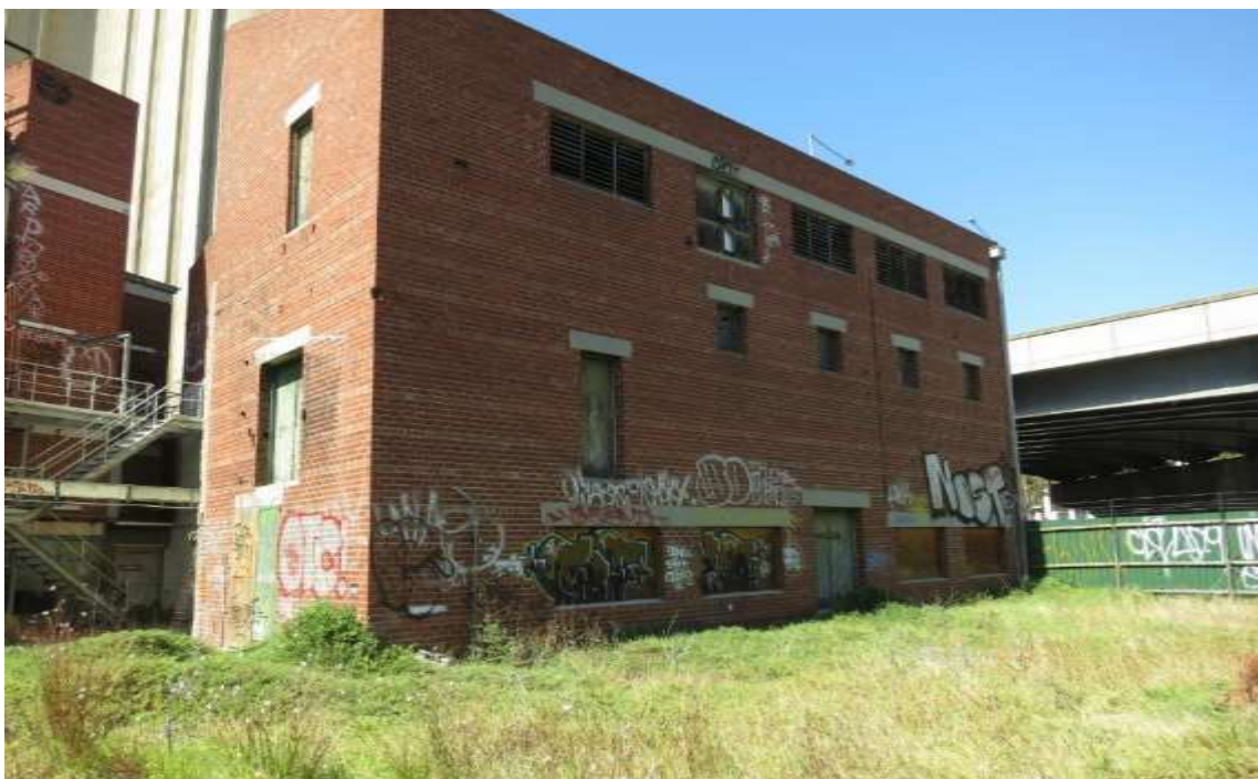
Figure 42 Another view of the west side of B11
