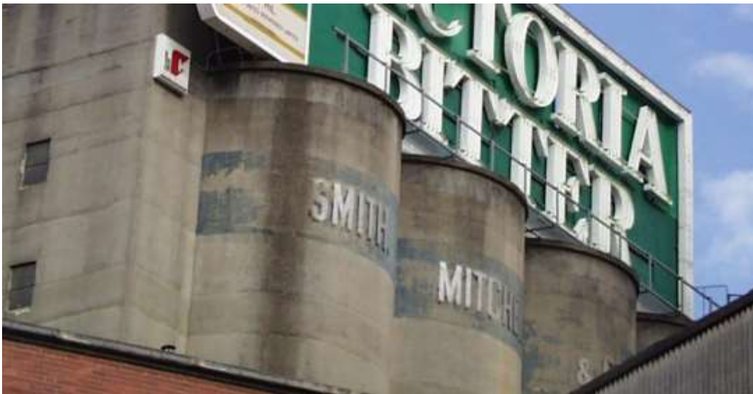
Figure 33 Detail of signage on west side of B8
