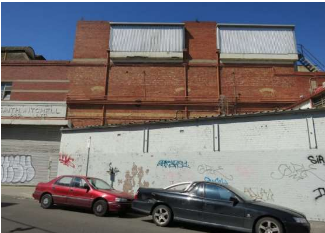
Figure 13 B5, north elevation to Gough Street; powder coated aluminium louvred screens will replace the corrugated steel panels to the north roof elevation; the painted wall to the 1918/19 north addition, in the foreground, will be retained but modified with new openings, and the paint removed
