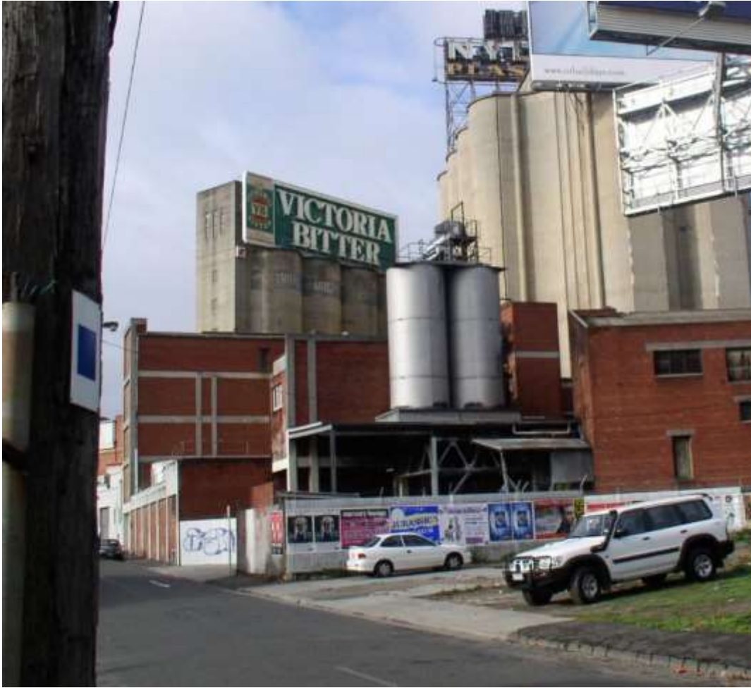
Figure 32 West view of B8 silos, with visible signage; B10 sits in front of the silos in this image.
