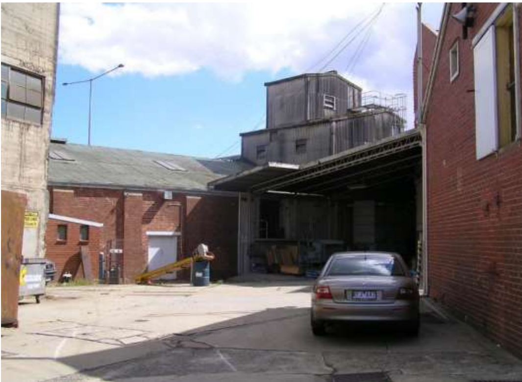
Figure 25 B6, another view of the north side of the building
