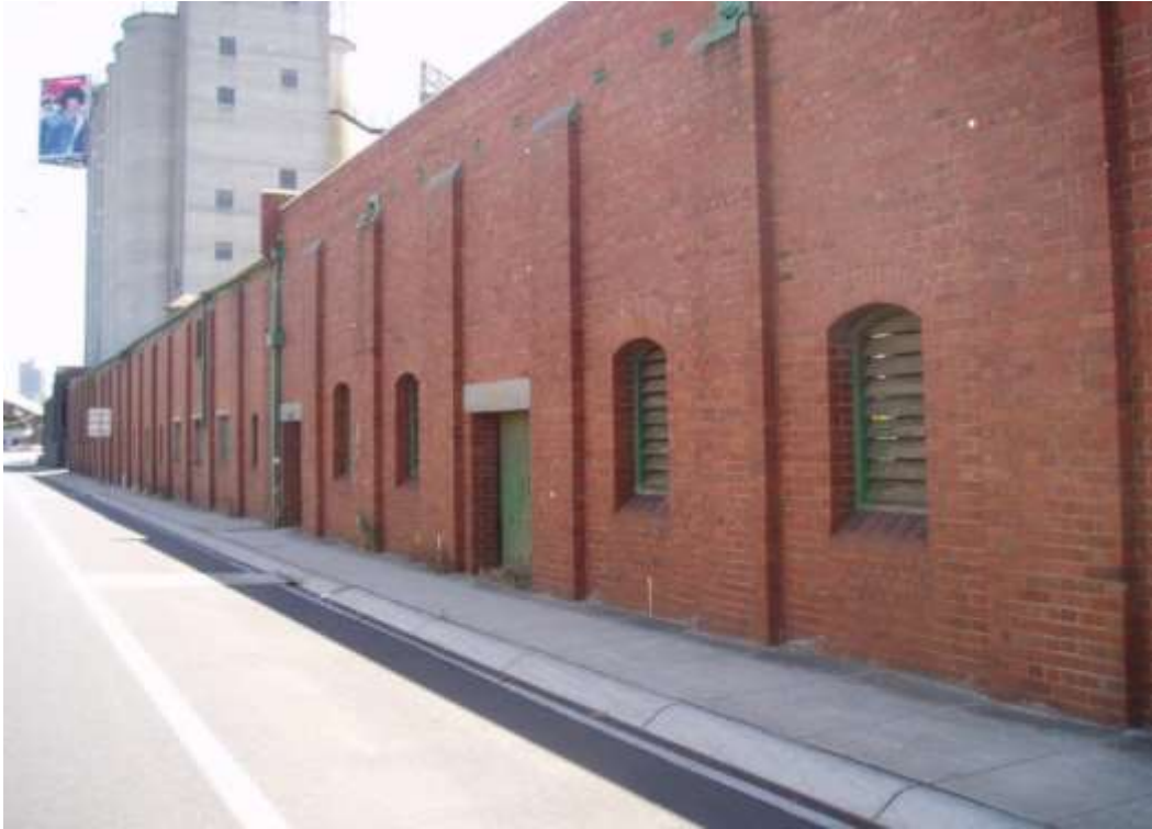
Figure 22 B6, south elevation to Harcourt Parade, with the wall of the 1928 east addition at right; this elevation will be retained
