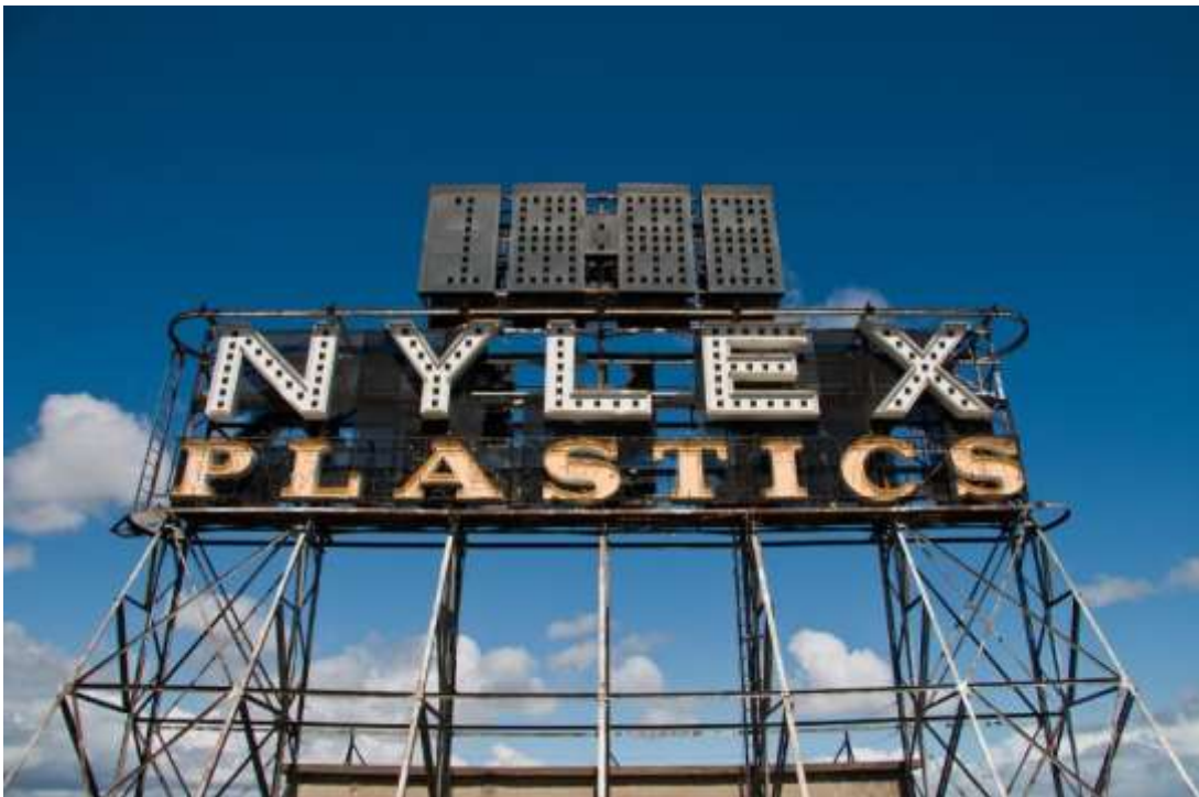
Figure 49 Detail of Nylex sign
