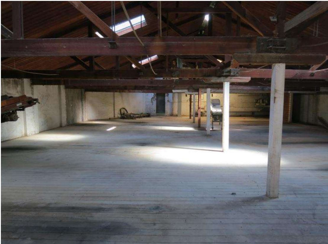
Figure 27 B6 interior, first floor
