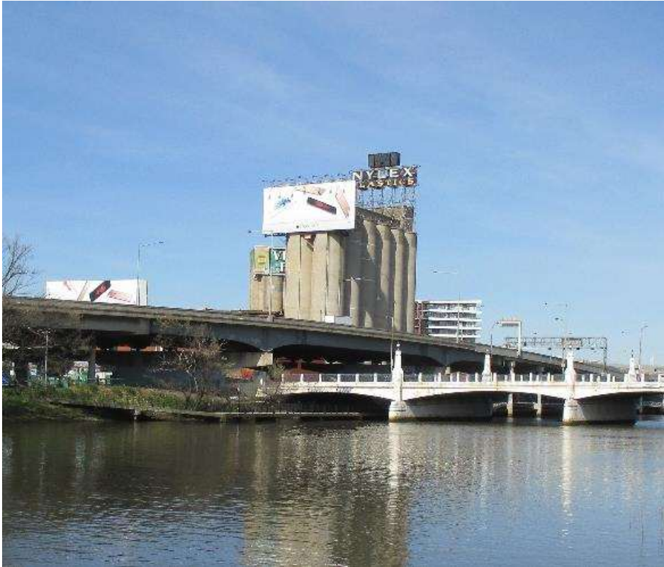
Figure 34 B9 silos, viewed from the south-west
