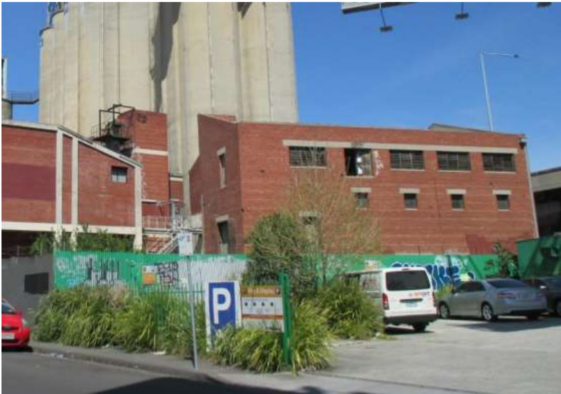
Figure 41 West elevation of B11 (at right); B10 is at left
