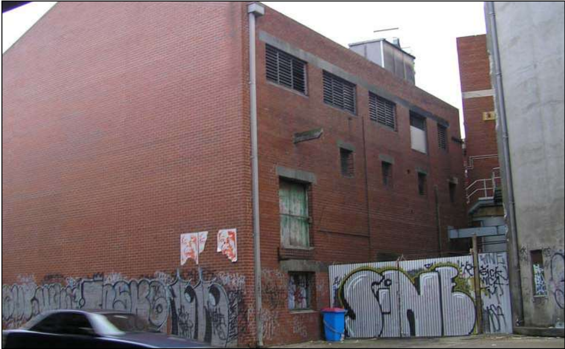
Figure 43 B11, non-original south elevation at left, and east elevation at right (as seen from Harcourt Parade)
