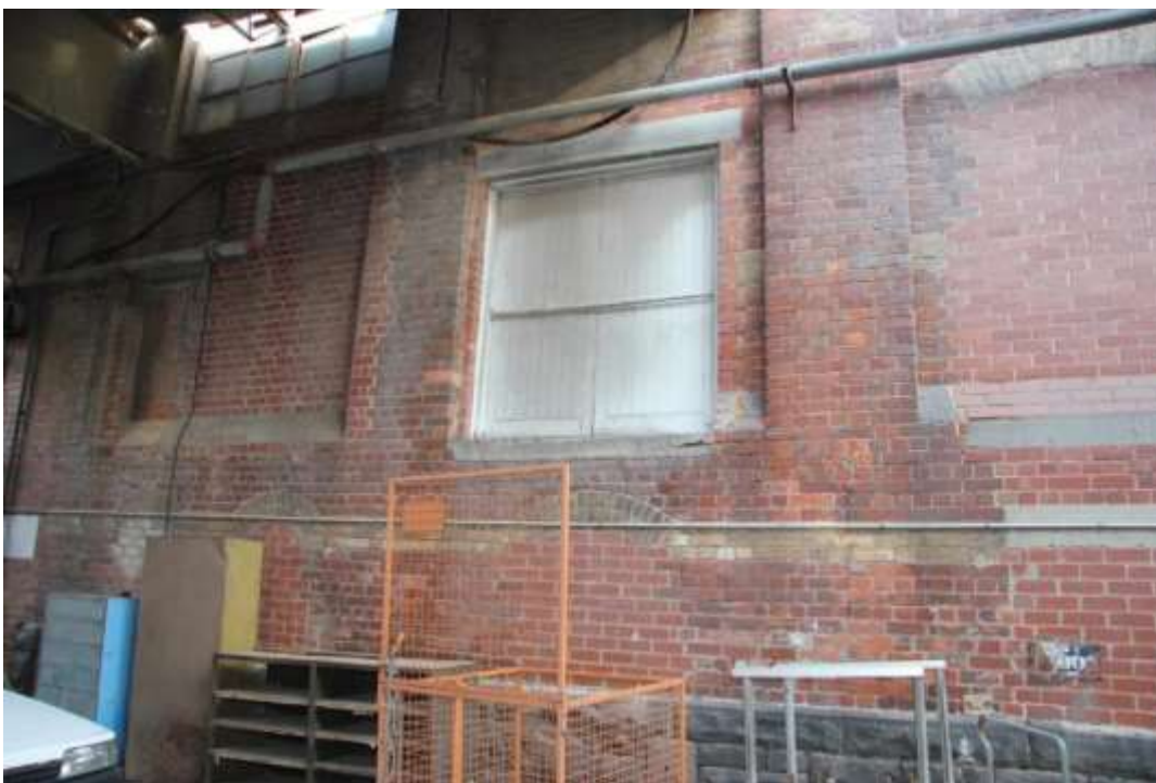
Figure 15 B5, east elevation
