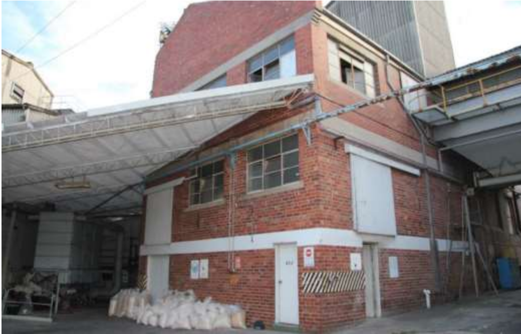
Figure 14 B5, south end, showing 1930s extension; the steel awning at left will be removed; the ground floor level walls will also be substantially removed
