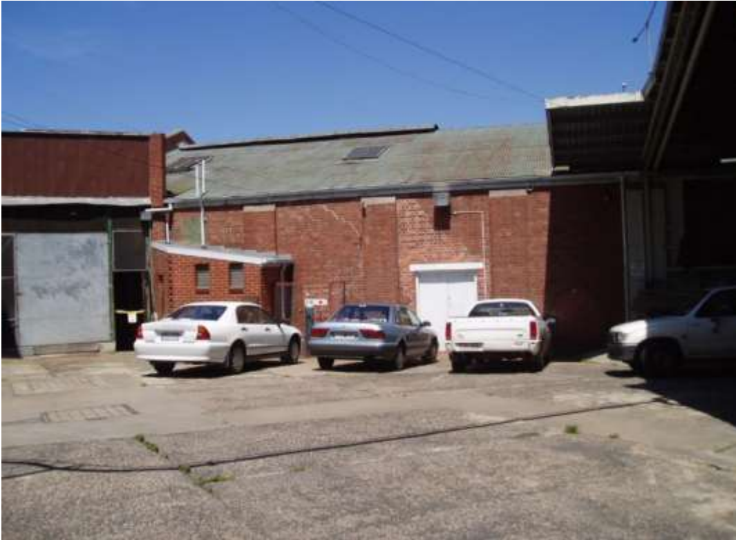
Figure 24 B6, east end, showing section of north wall and roof; this building component is being retained, excluding the addition at left and the adjoining minor brick annex
