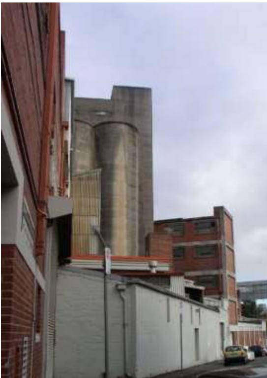
Figure 31 North end of B8 silos, as seen from the east
