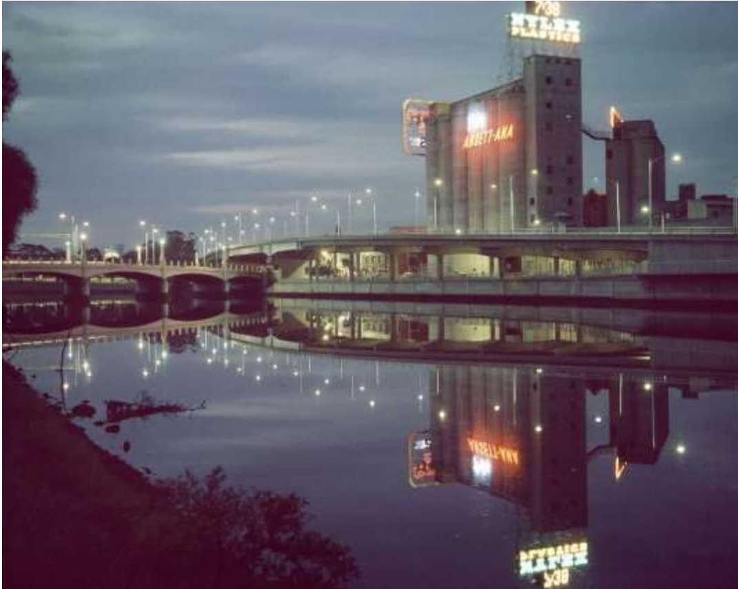
Figure 46 C. late 1960s image, showing the completed silos and Nylex sign, plus other signs which have subsequently been removed/replaced Source: State Library of Victoria
