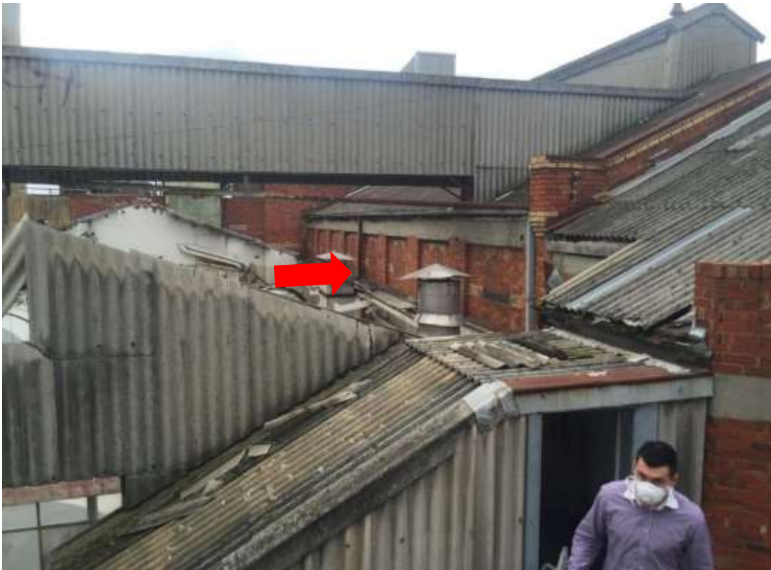
Figure 16 View to top level and roof of B5, showing part of the original 1880s bichromatic brick west elevation (indicated)
