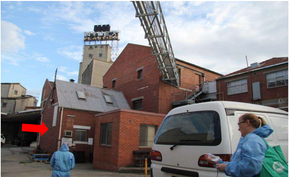
Figure 10 B4, south end; the south bay (as indicated) is proposed for removal with the Stage 1 permit application; the building at right is the rear of B3
