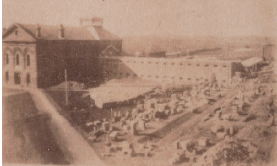
Figure 1 Photograph showing the south wing of A Division under construction, c1896. Source: State Library of Victoria Online Picture Collection, 'Scenes from Pentridge', Accession No. H96.160/509.
