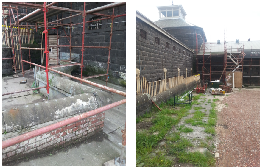
Figure 10 The photograph on the left shows the dwarf wall earmarked from demolition, while the photograph on the right shows the fence to be retained.
