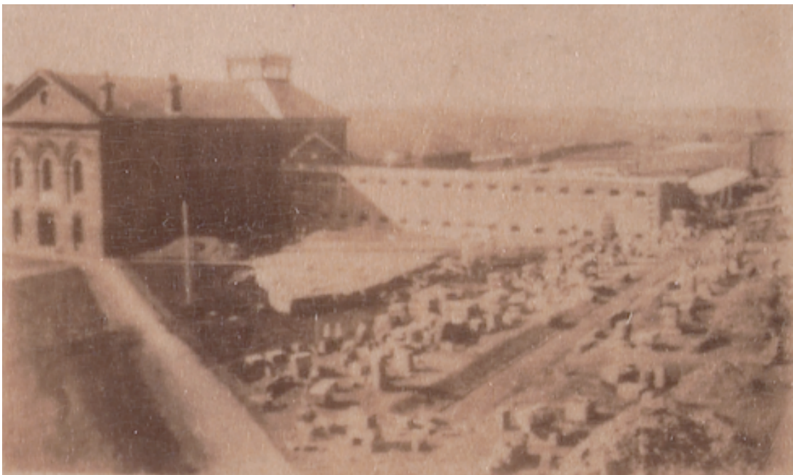
Figure 25 Photograph showing the south wing of A Division under construction, c1896. Source: State Library of Victoria Online Picture Collection, 'Scenes from Pentridge', Accession No. H96.160/509.
