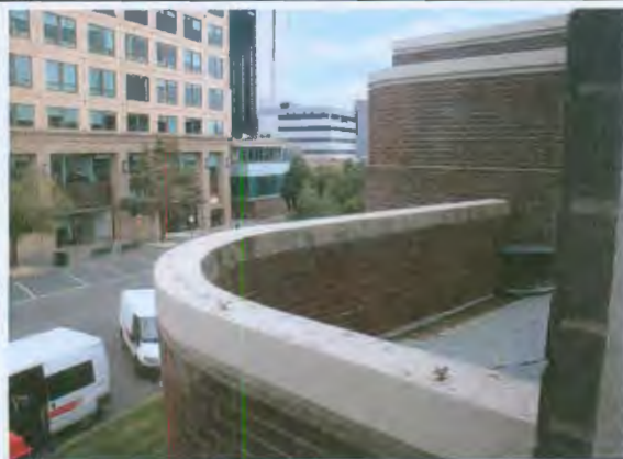
View to parapet on southern façade concealing corrugated metal roof.
