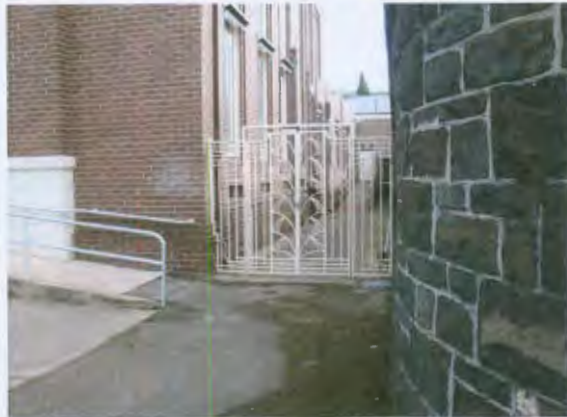
Decorative wrought-iron gates.
