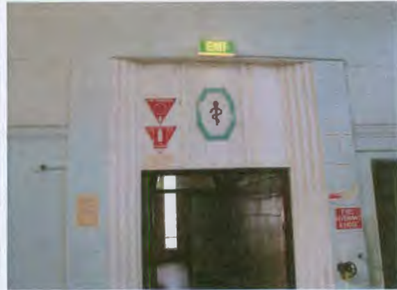
Decorative internal wall mouldings and art deco detailing.
