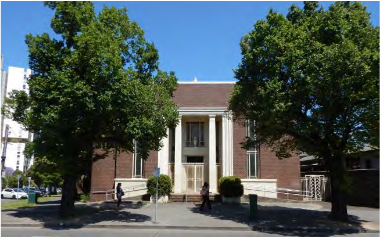
Plate 1. Entrance to building, St. Kilda Road (Facing west)
