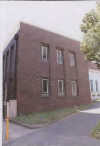
Photograph 5: 1947 addition Coventry Street frontage. (Source: Biosis 2016)
