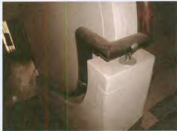
Turned timber hand rails to stairs.
