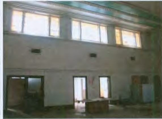
Steel framed ribbon windows and decorative ceiling mouldings.
