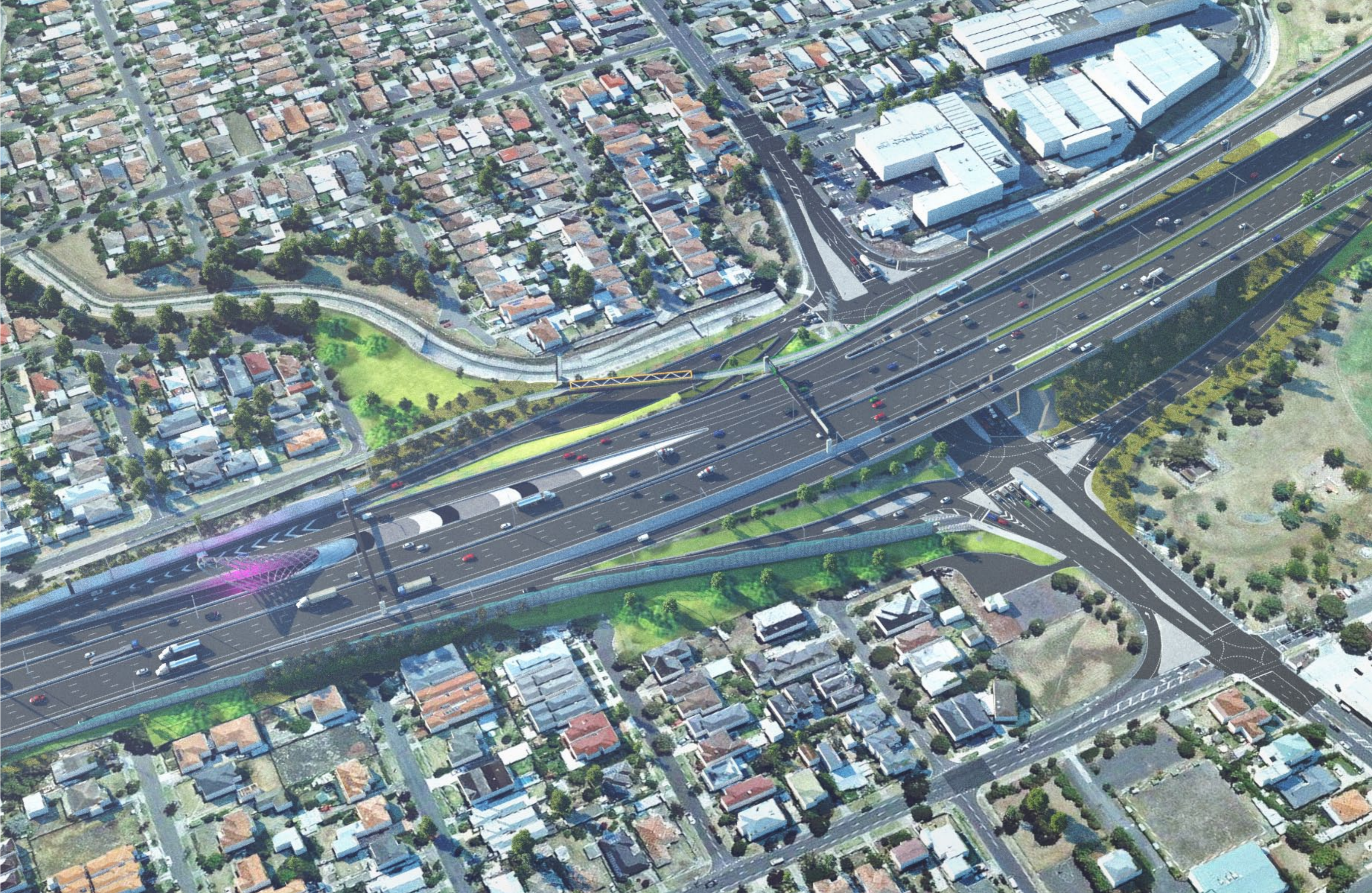
SOUTHERN ENTRY PORTAL VICINITY
