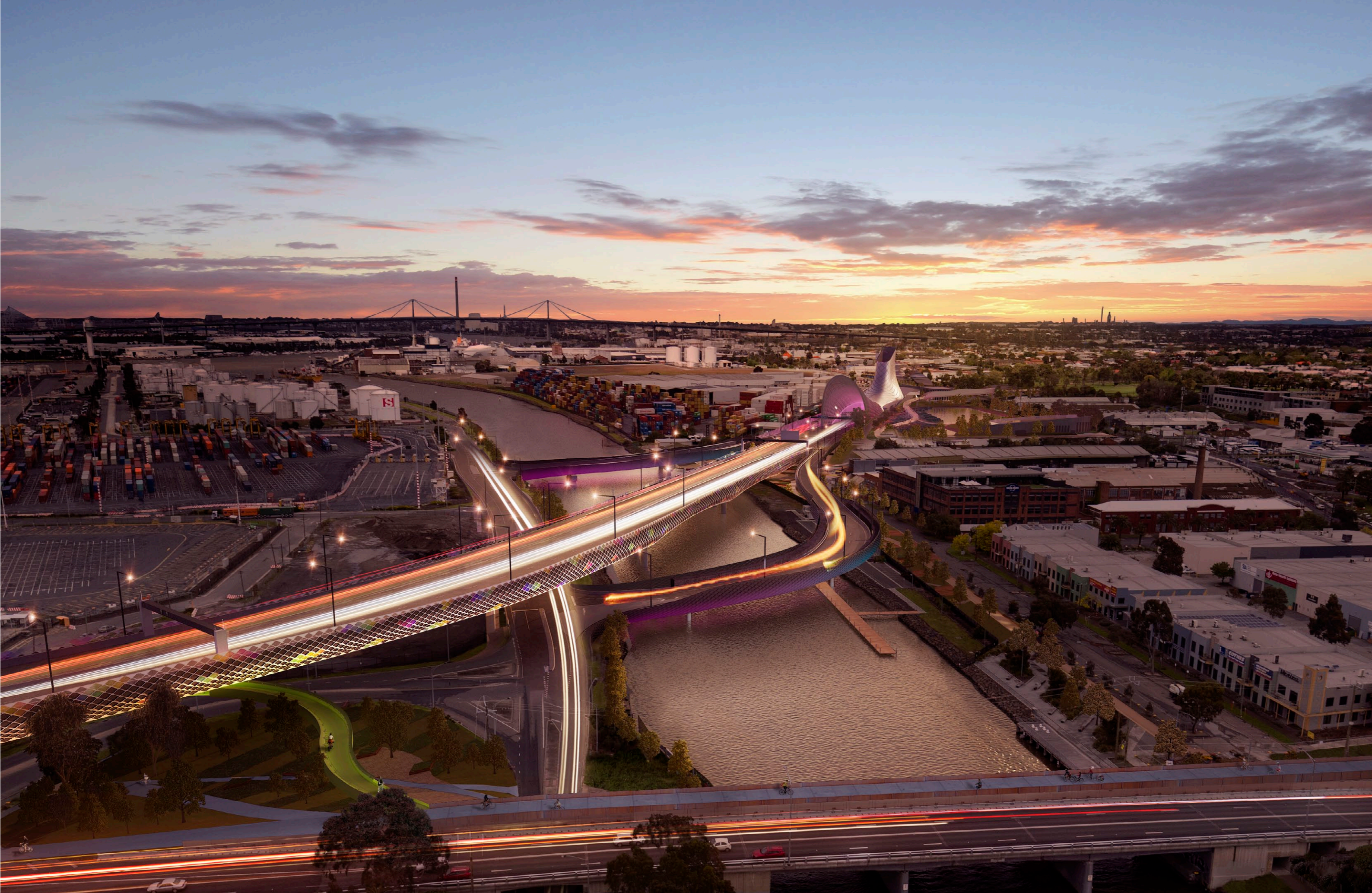
AERIAL OF MARIBYRNONG CROSSING NIGHT VIEW
