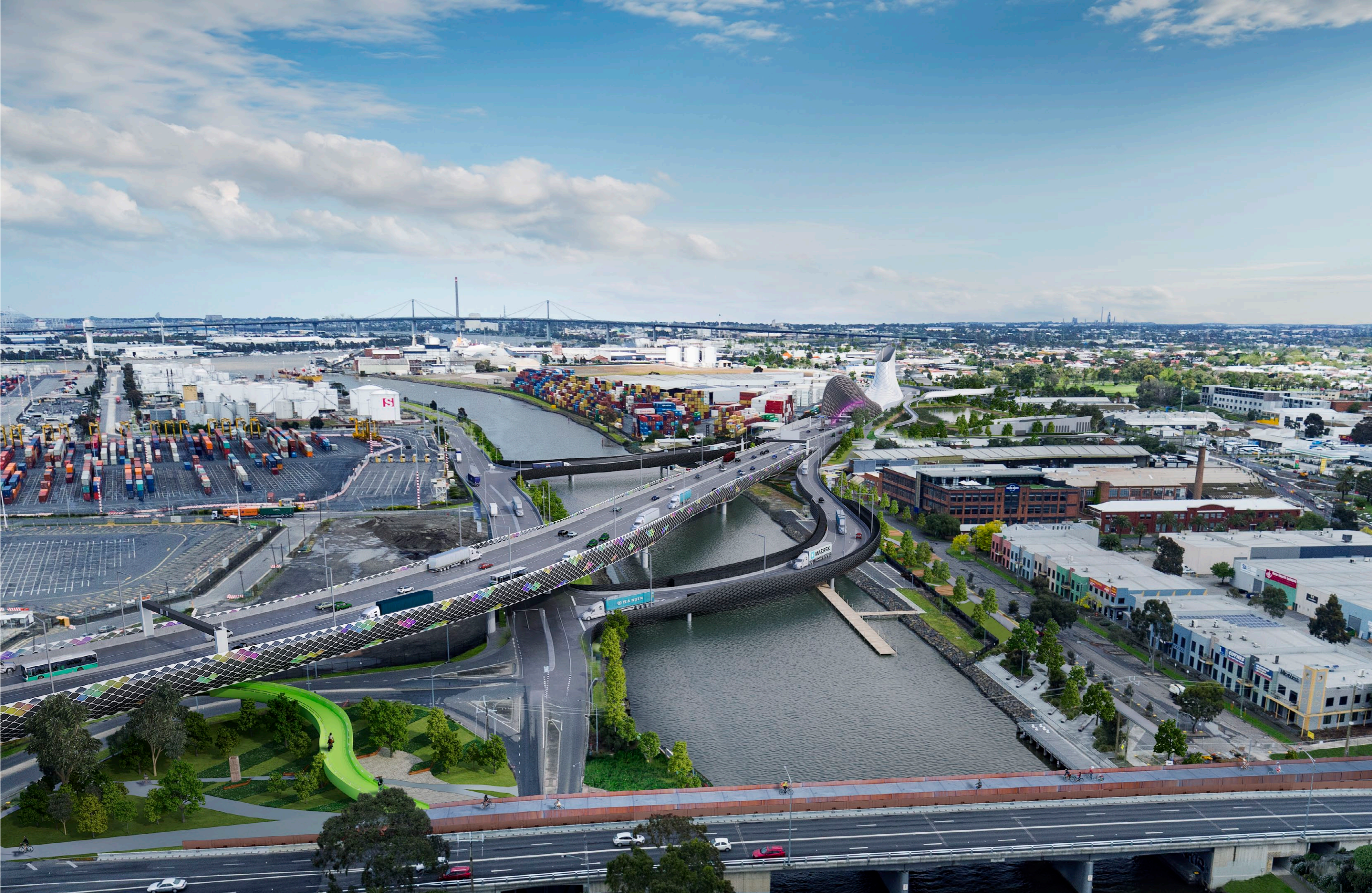
AERIAL OF MARIBYRNONG CROSSING
