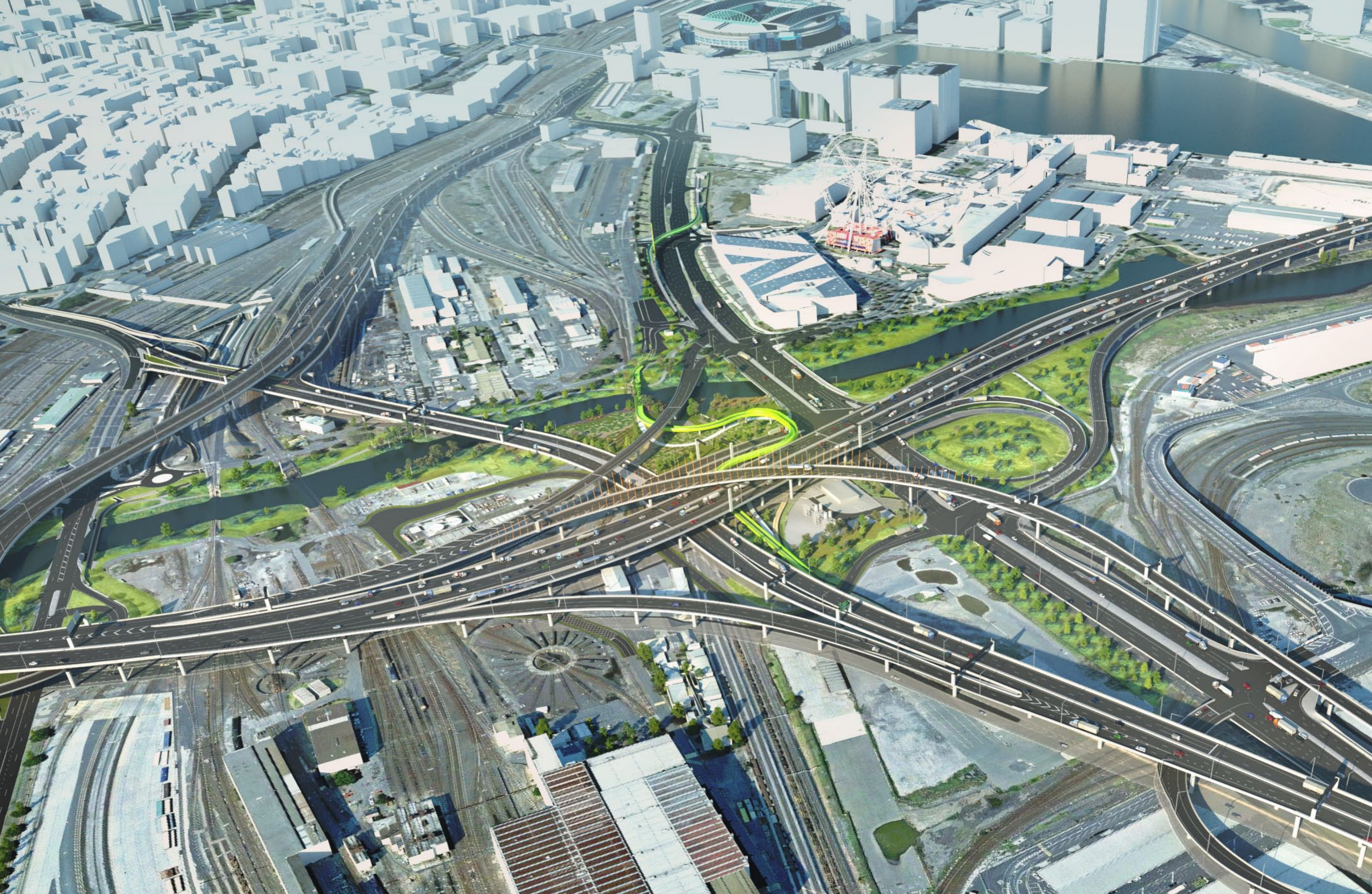
CITY CONNECTION AERIAL VIEW
