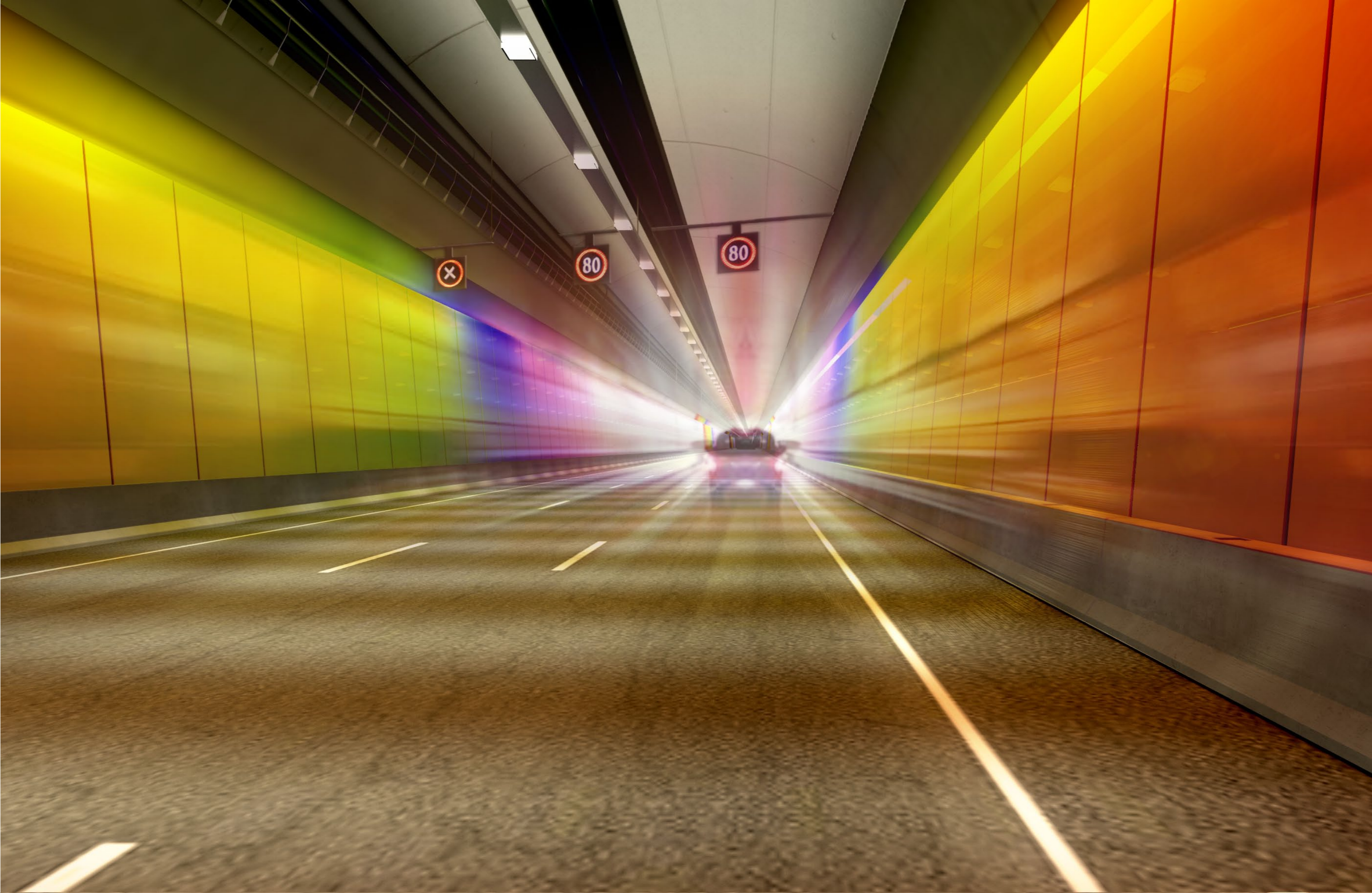
VIEW OF TUNNEL
