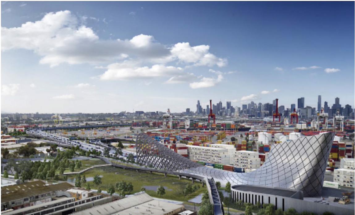
Aerial view of northern portal and ventilation structure, facing north-east
