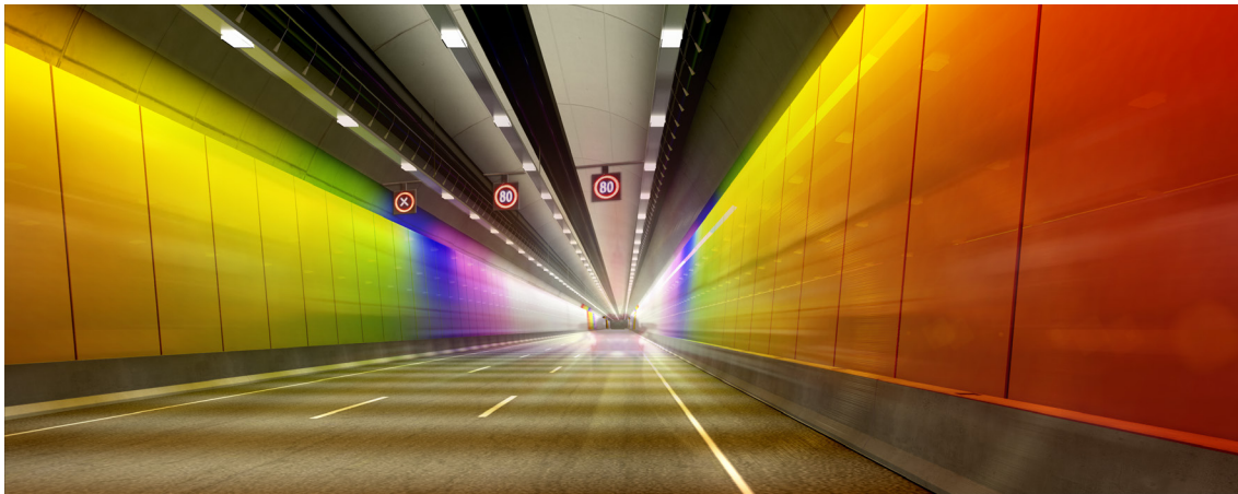
Figure 6-9 Driver view of tunnel interior
