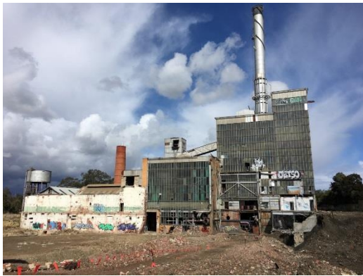
Figure Two: North elevation, August 2016, source: Heritage Victoria
