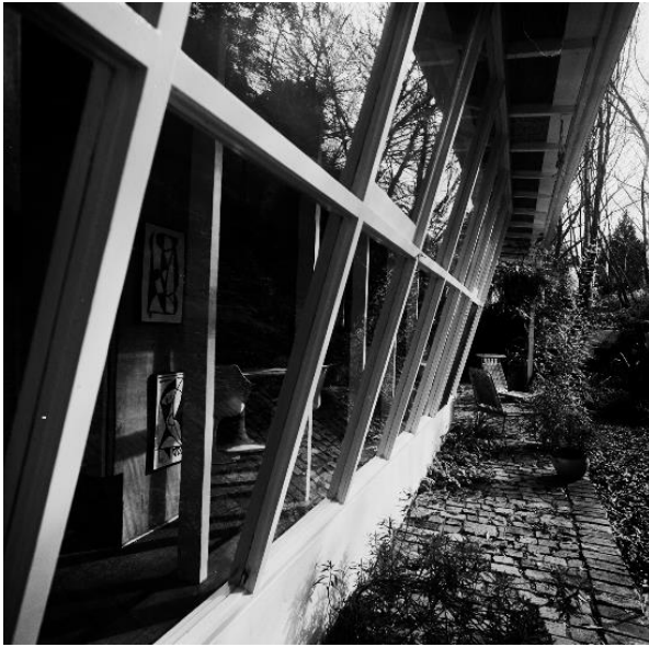
Left: 1947, Canted windows to the living area, showing the structural studs internally.
