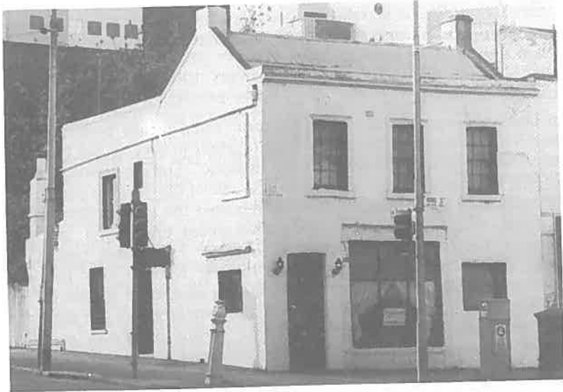
This 1850s corner shop, a rare relic of Melbourne's earliest phase of development, earned a place on the State's Historic Buildings Register, largely for its relative antiquity in a part of the city now dominated by high-rise office buildings. (Photograph: VGPO)
